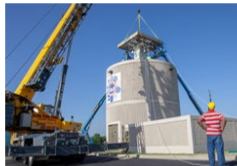
ATD Installation in Norman
