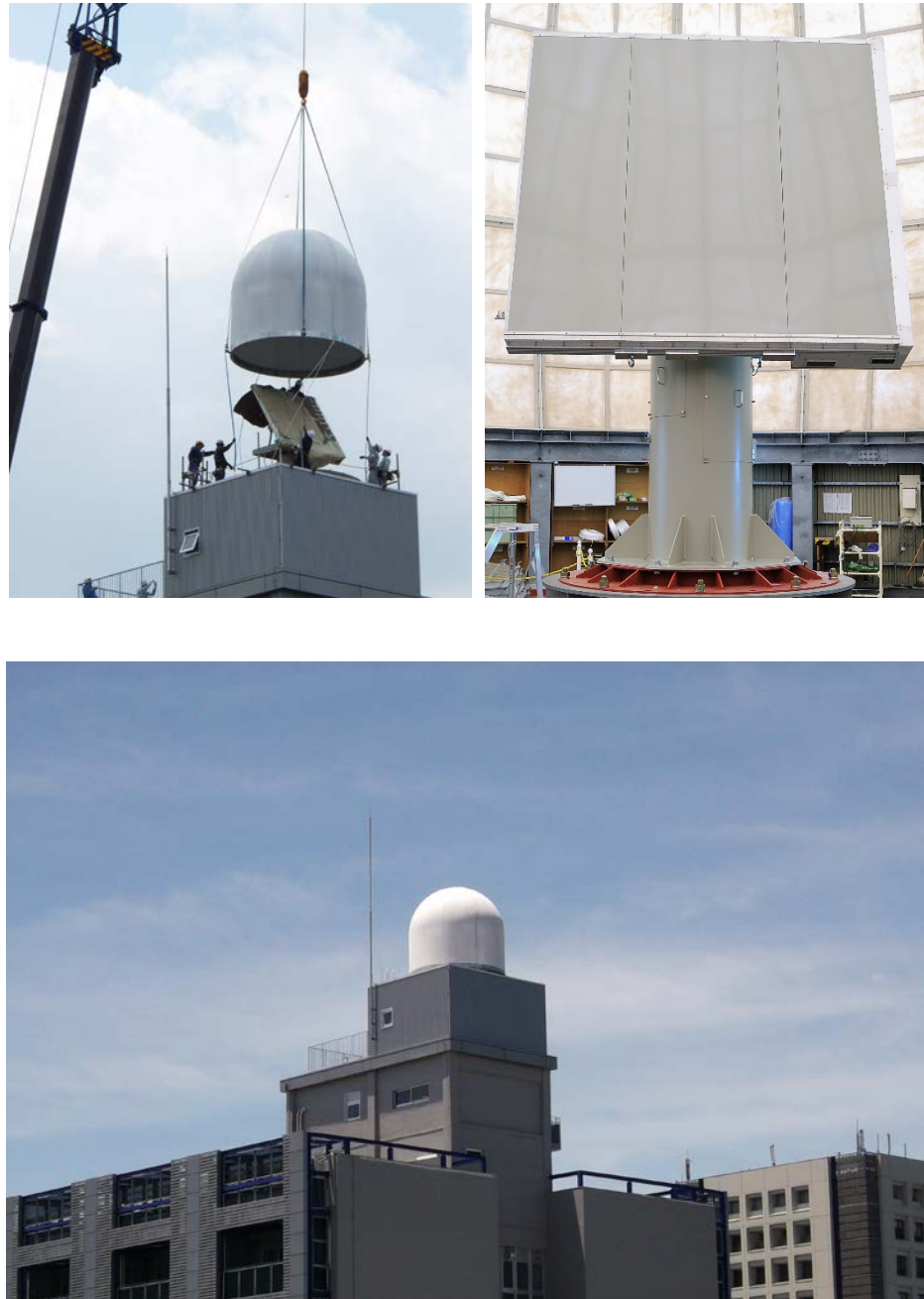
Fig. 1 Photographs of the Phased Array Radar (PAR) at Suita Campus in Osaka University. Top left panel shows the installation of the PAR in May, 2012. Top right panel shows the antenna of the PAR system inside the Radar Dome. Bottom panel shows the overview of the PAR at the Electrical, Electronic and Information Engineering Department building in Osaka University.
