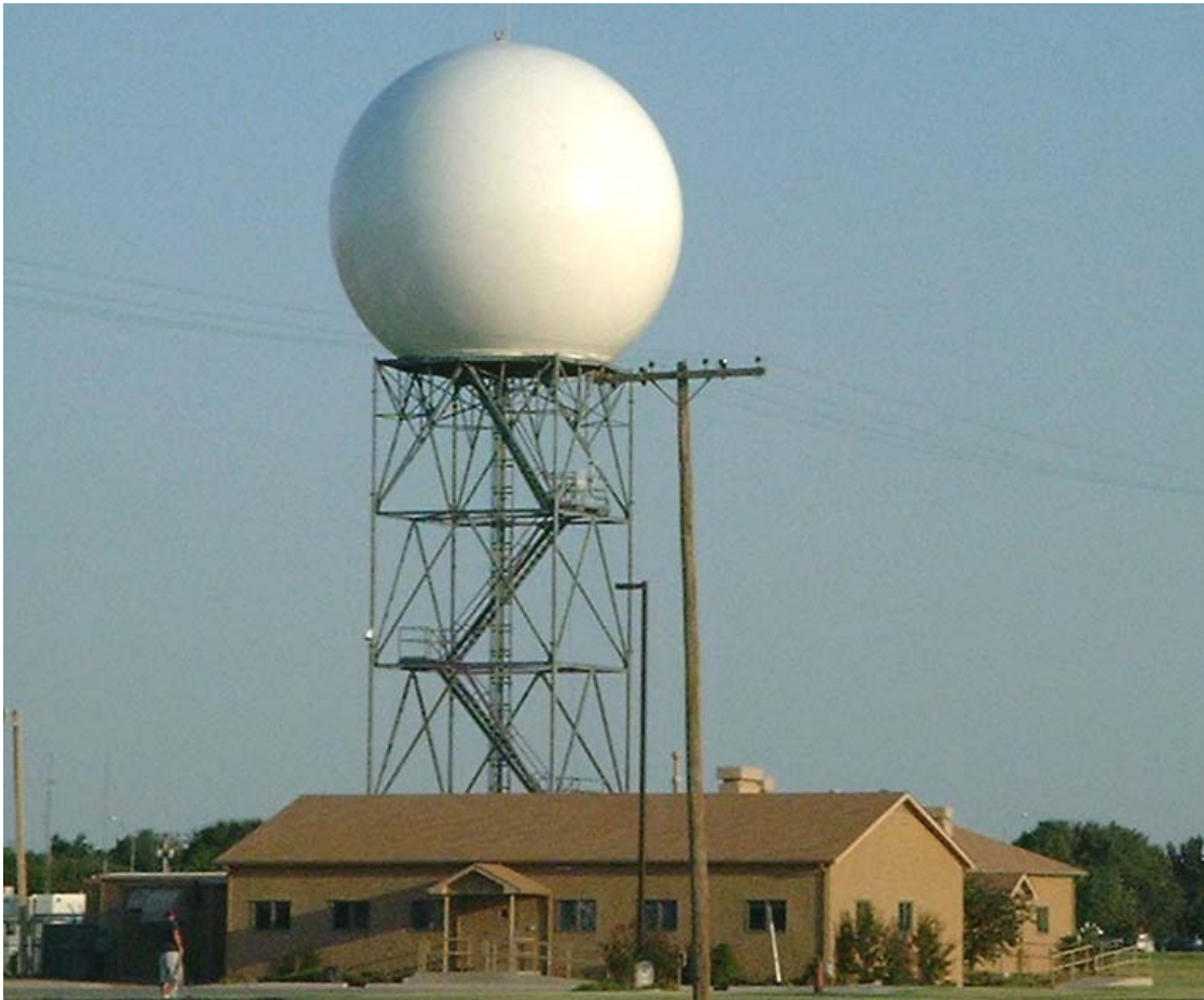
Figure 2.1: KOUN Doppler Radar WSR-88D used for data collection in this work.
