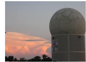
Phased Array Weather Radar
