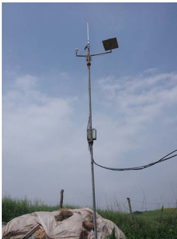
Fig. 1 The Antennas of LMS
