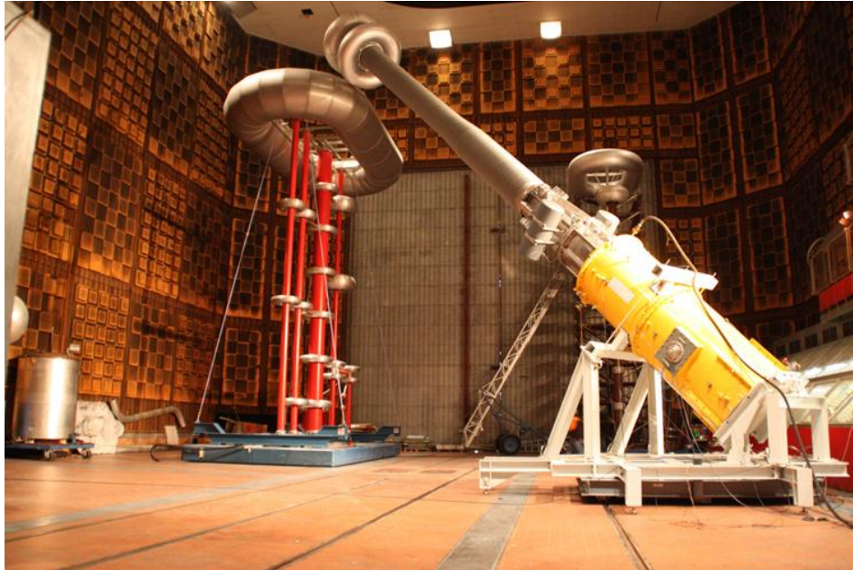
Photo 10: DC test of transformer bushing, Graz University of Technology
