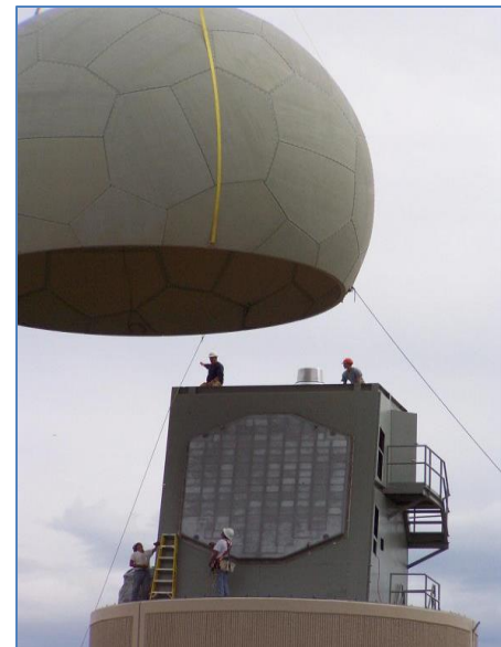
Figure 3: The Navy SPY-1A antenna is installed in the NWRT/PAR facility at Norman, OK in 2003.
